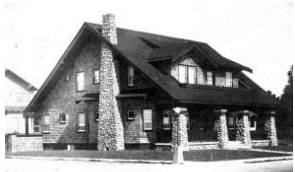
River rock and wood shingles help define this Craftsman-style home on Alameda's East End. Photo: alamedainfo.com
